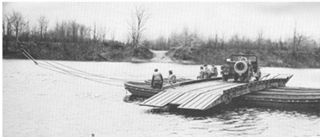
Light tactical raft is constructed by members of the 175th Engineers
