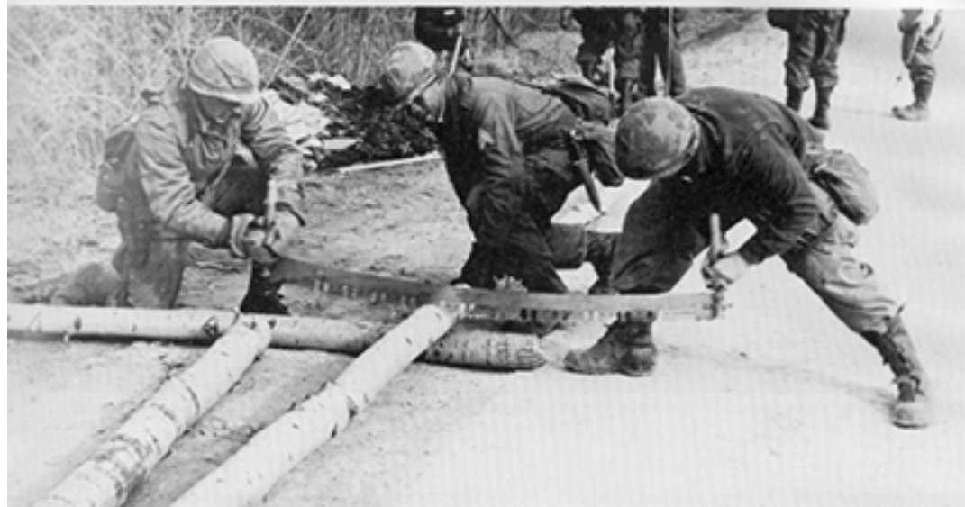
175th Engineers build protective cover for a culvert.
