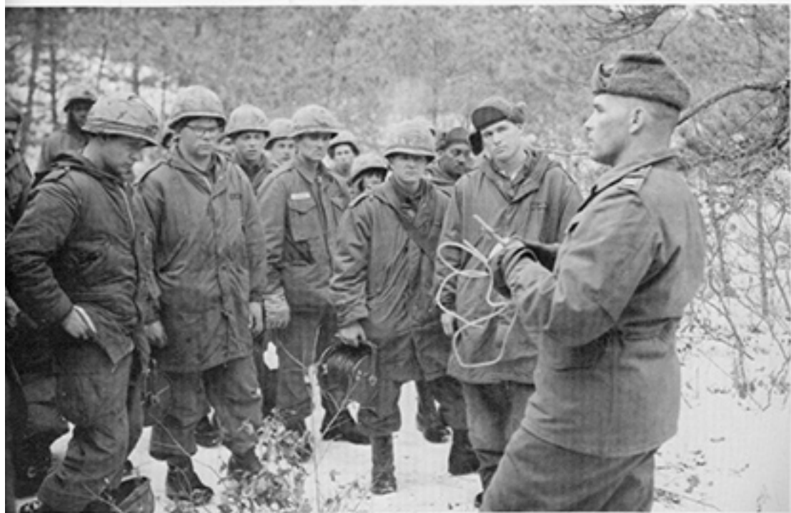
Capt. Stearns, C.O. of 175th Engineers instructs in demolitions
